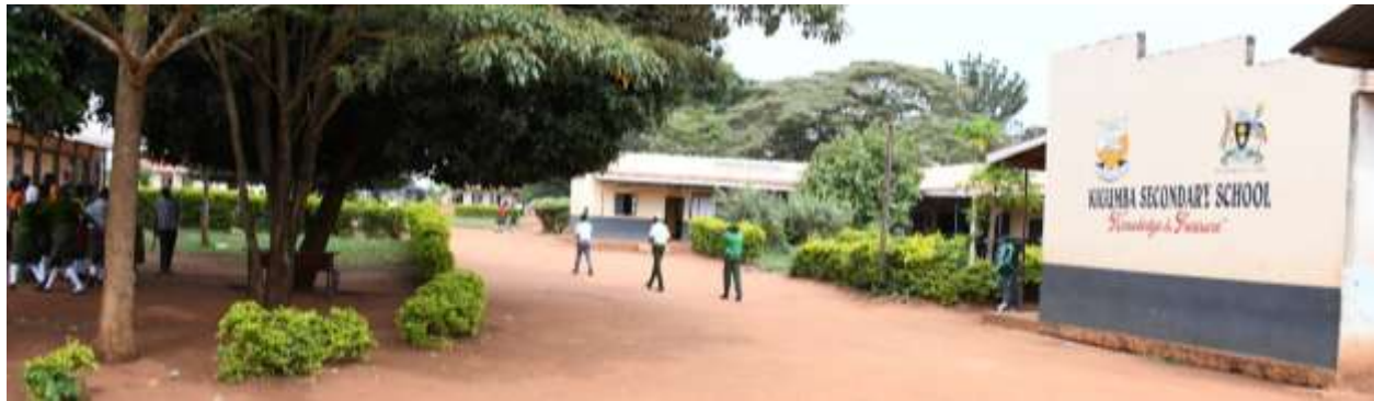
Some of the existing classrooms constructed by PTA at Kigumba SS
